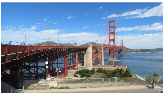
Golden Gate bridge
